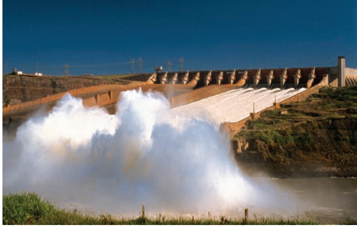
The Itapu dam in Brazil is the world's largest provider of hydro-electricity.
